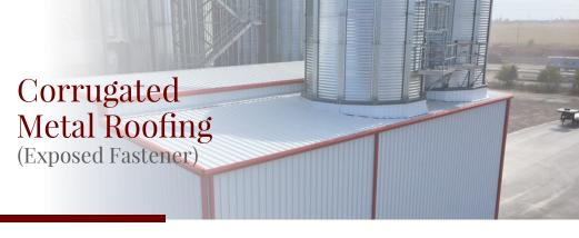
The second style of metal roofing is exposed fastener roofing, also called corrugated metal roofing. As the name suggests, the main difference in this roofing style is that the metal is attached to the roof with exposed screws.
